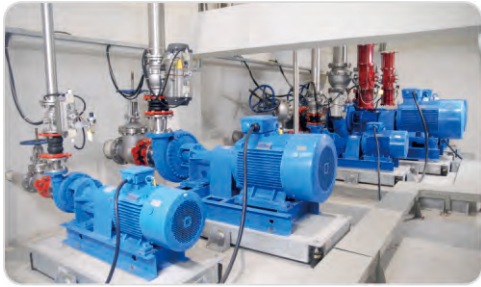
PUMP equipment (The maximum horsepower is 110KW per unit)
